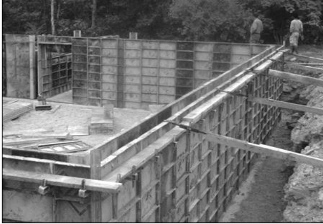
Figure 10. Metal framework with plywood sheathing faces
