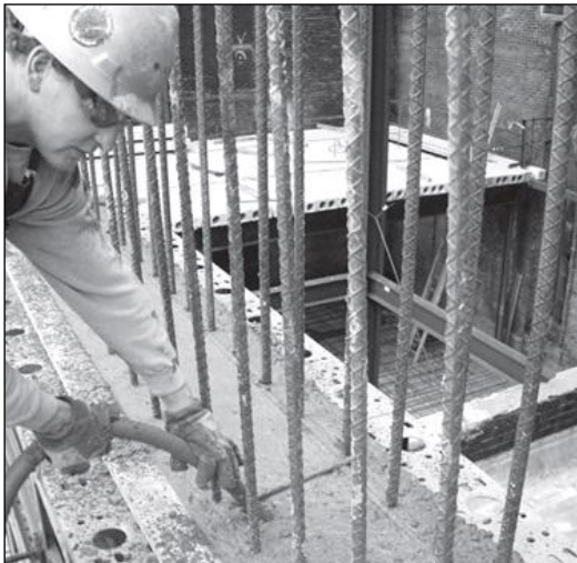
Figure 8. Vibration of concrete
