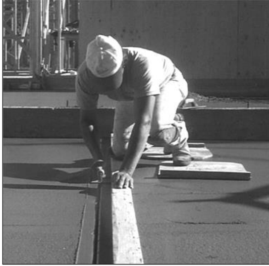
Figure 6. Grooving of concrete slab
